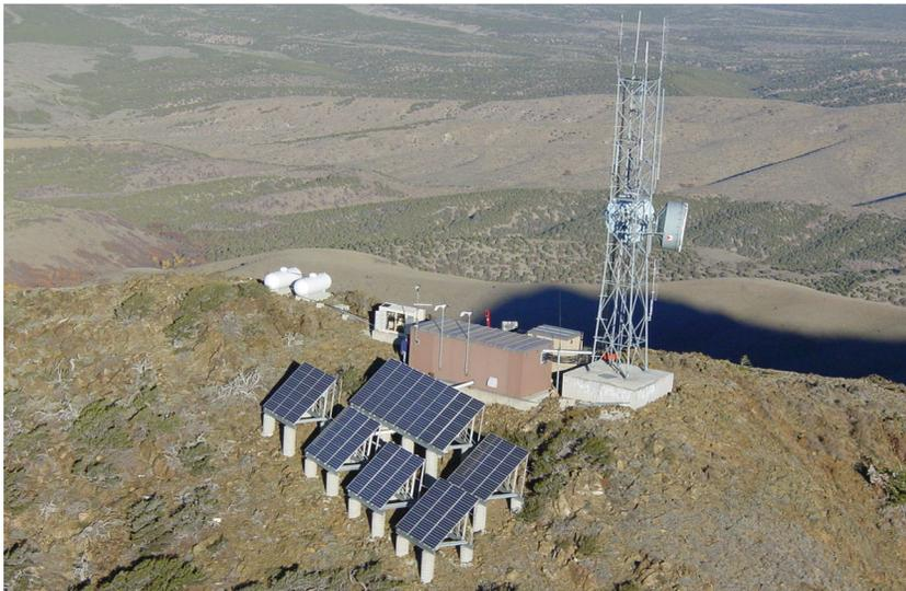
From a 9400-foot mountaintop, the last hop in Tooele County's Emergency Management System backhaul covers the vast western desert of the 7000-square-mile county. Run on solar energy with generator backup, Eclipse Packet Node IRU 600 has better power usage characteristics compared to its TDM predecessors, sparing EMS costly maintenance trips via helicopter.
